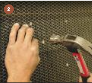
Install corrosion resistant metal lath.
