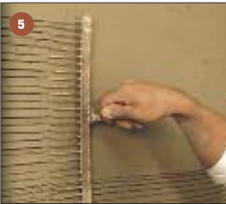
Rake mortar to create scratch coat. Allow to Dry.
