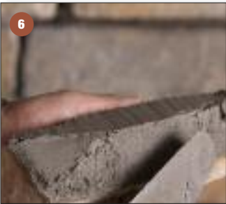
Apply mortar to the entire back of the stone.
