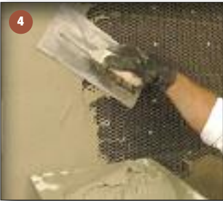
Apply mortar for scratch coat.
