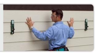
Working as a pair, the Gecko Gauge clamps to each siding course, acting as a second set of hands to gauge and support the next course for nailing. Get fast, accurate installation with less fatigue and with virtually no layout.
